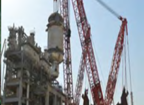
WIDE AFFILIATES REPLACEMENT OF EO REACTOR
