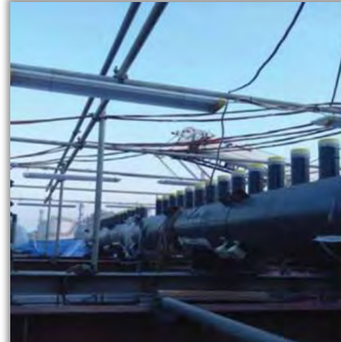
Refractory Lined Outlet Header (RLOH) Replacement At SASREF
