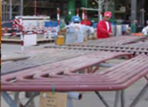
RE-TUBING OF 8-UNIT ETHYLENE FURNACE AT UNITED
